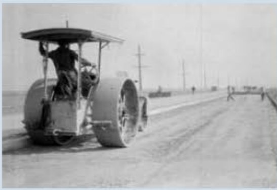
1930s: A form of RCC paving is performed in Sweden.
