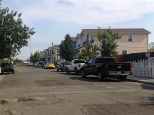
Hickory Street with current asphalt surface
