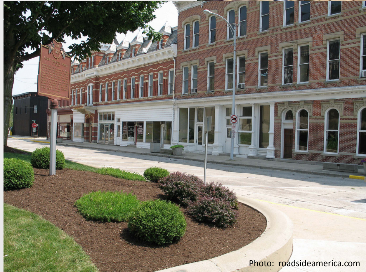
Bellefontaine, Ohio – 125 Year Old Concrete Pavement
